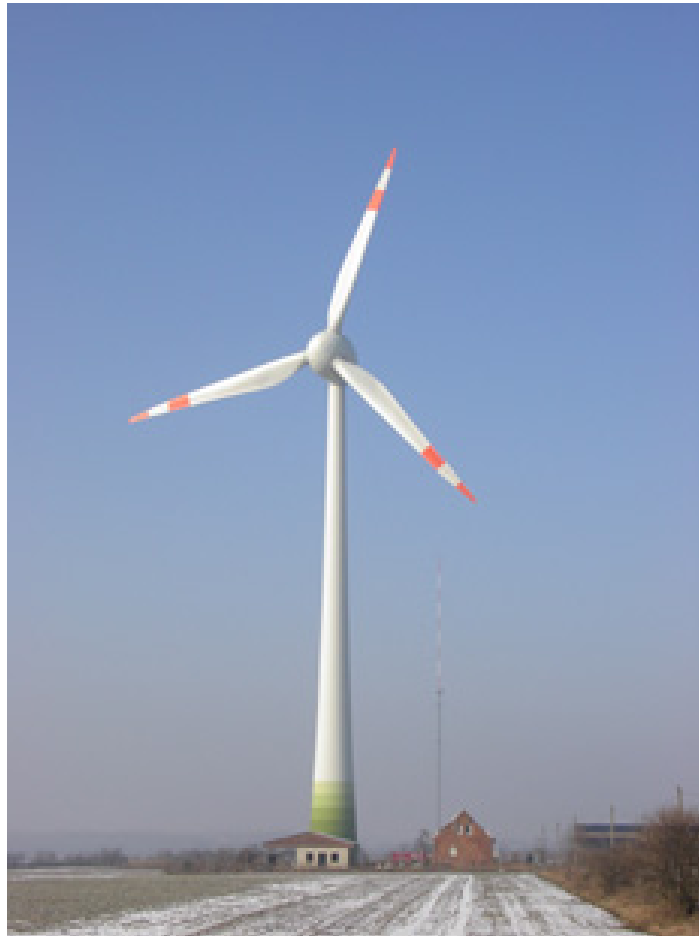
Fig. 4.4: Enercon 112 with a capacity of 4.5 MW
