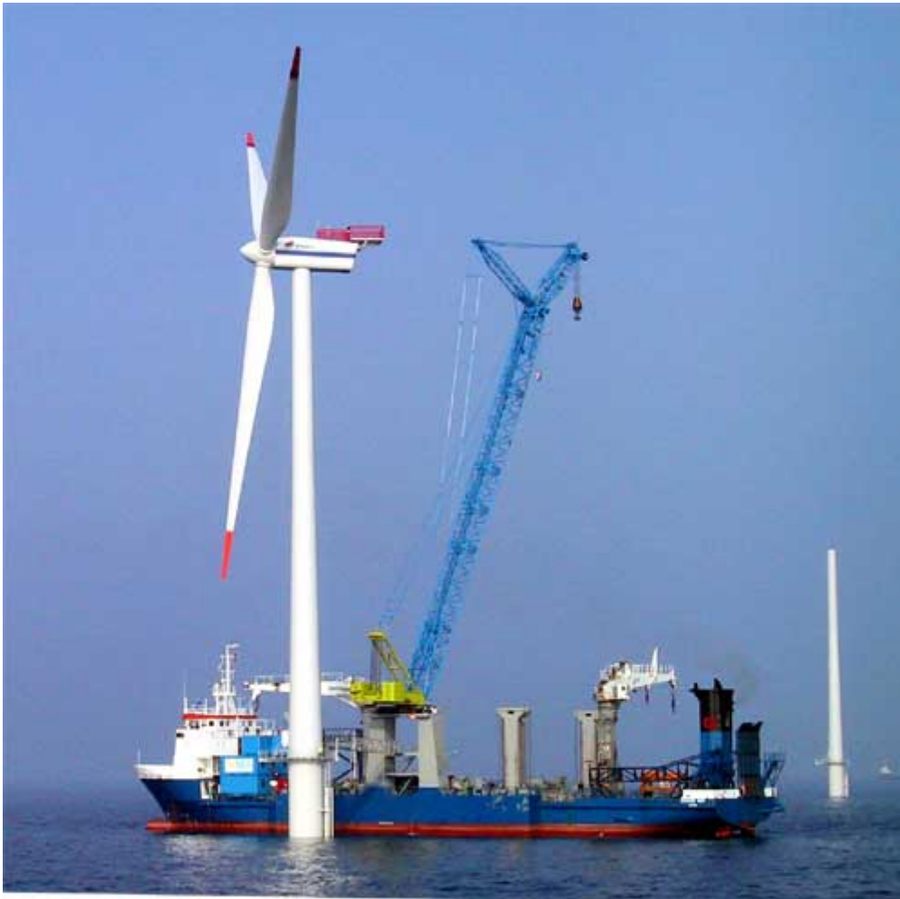
Fig. 4.22: A2SEA, example of modified hoisting vessel for installation and maintenance of offshore wind turbines
