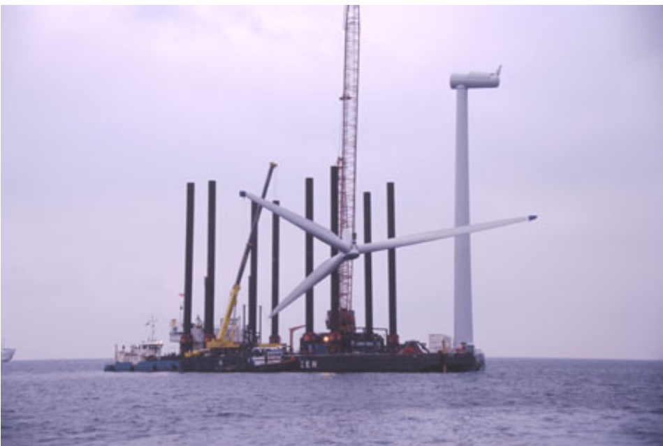
Fig. 4.10: Entire rotor being assembled
