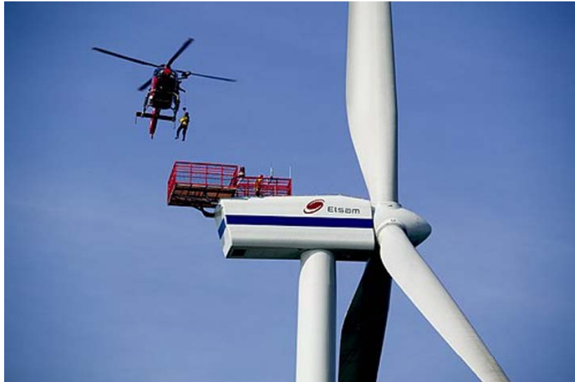
Fig. 4.15: Hoisting personnel onto a turbine
